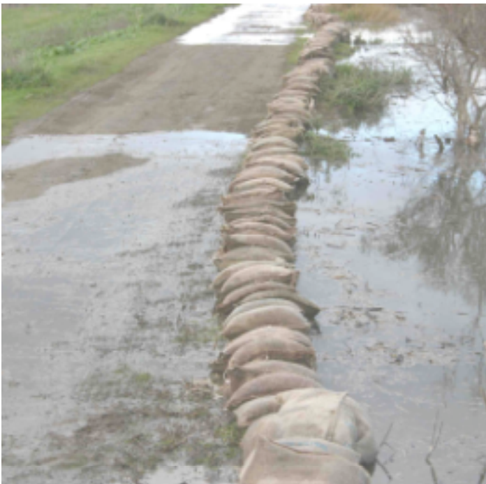
Sandbags hold tide at levee across from tower.
